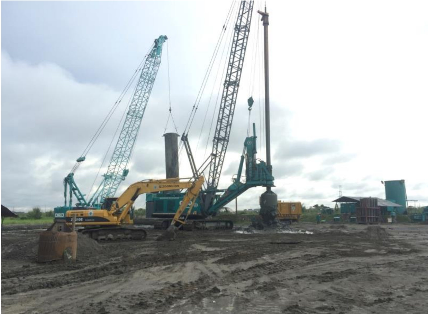
Bored piling foundation works on site
