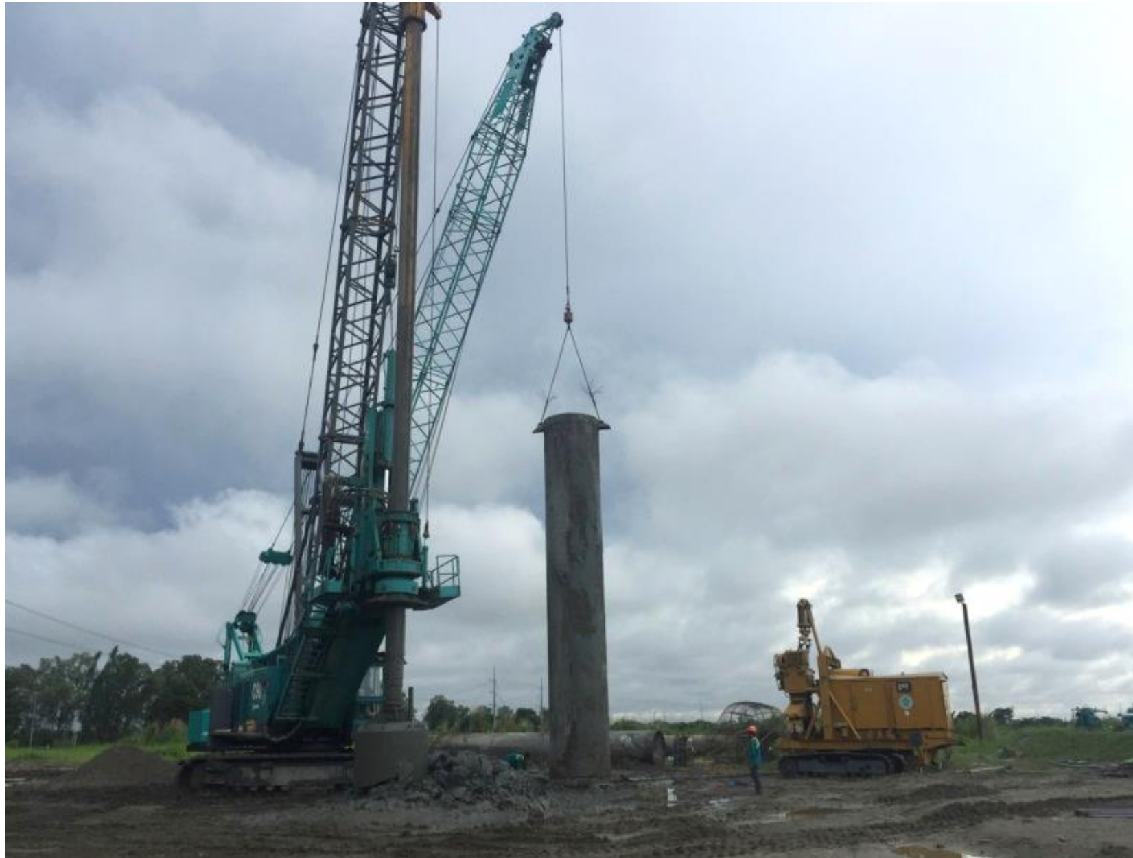
Bored piling foundation works on site
