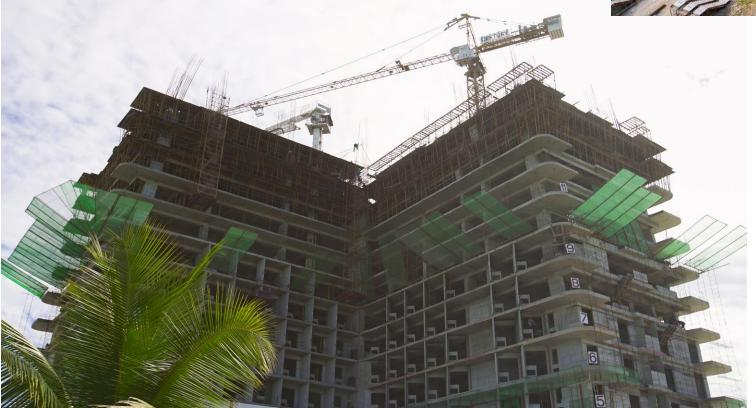
Installation of pre-cast partition of balconies is on-going and already at 9th floor
